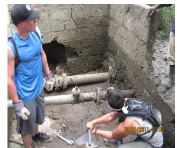
Community water system repaired!
